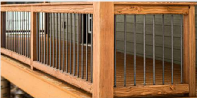
4x4 Railing with Rebar
